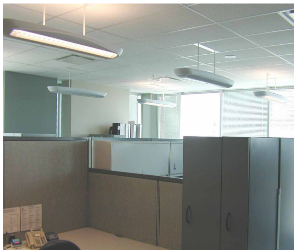
Figure 2 Ergolite's occupancy sensors save energy by turning off desktop lights over vacant spaces
