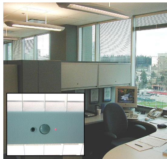
Figure 1 Ergolite lighting system – included occupancy and photo control sensors in detail
