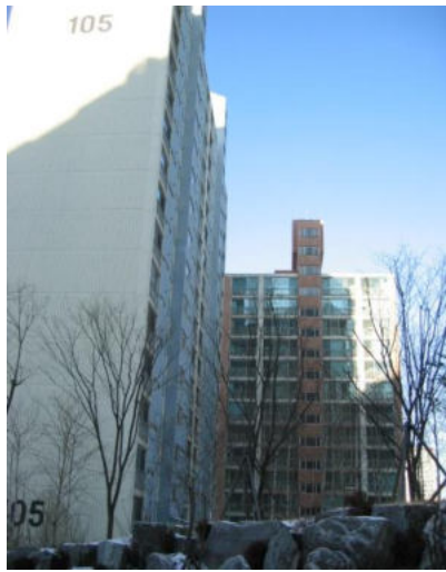
Photo 1 Building 105 of J Apartment House
