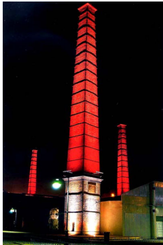
Figure 5 Example of an installation where LED-lines are placed against the lighted area itself.
